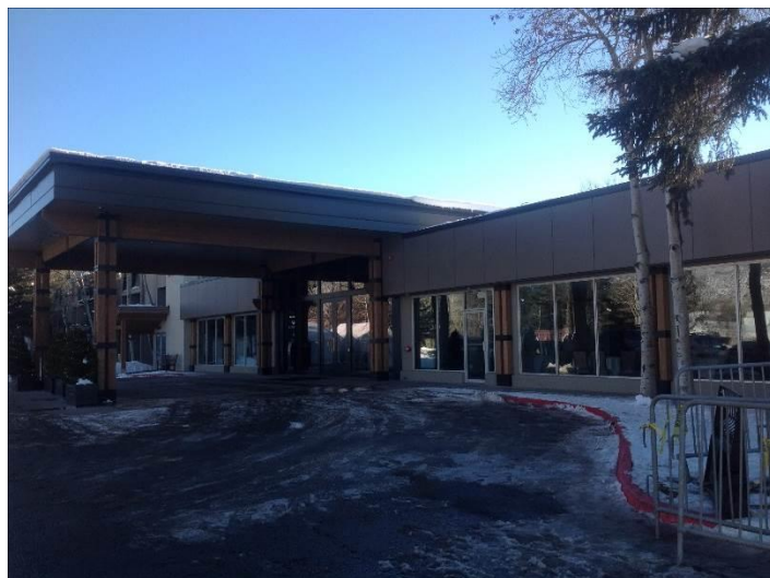
Approximately 5,000 sq. ft. of RevealShield UV Stable Water Resistive Vapor Permeable Air Barrier Membrane was installed on The Inn at Aspen at the base of Buttermilk Mountain in Aspen, Colorado.
